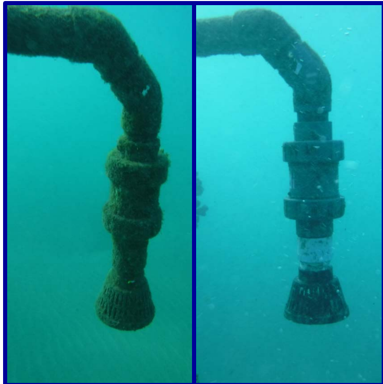
Above Left: The RO intake before cleaning, covered in bio-fouling.
